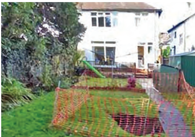
Collapse of the tunnels in the rear garden of 20 Iberian Avenue in 2014.
